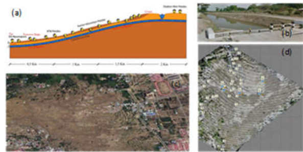
Fig. 11. (a) Model of The Collapse Mechanism of the Petobo Liquidation Collapse, (b) Gumbasa Irrigation Canal Before The Earthquake, (c) Image of Liquefaction Aerial Flow 16 Days After The Earthquake, (d) Aerial Contour Image
